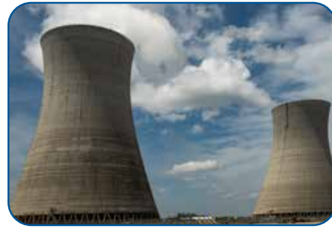
Vogtle 3 and 4 cooling towers
