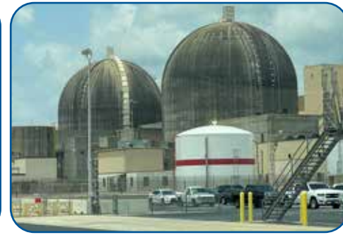
Vogtle 3 and 4 containment buildings
